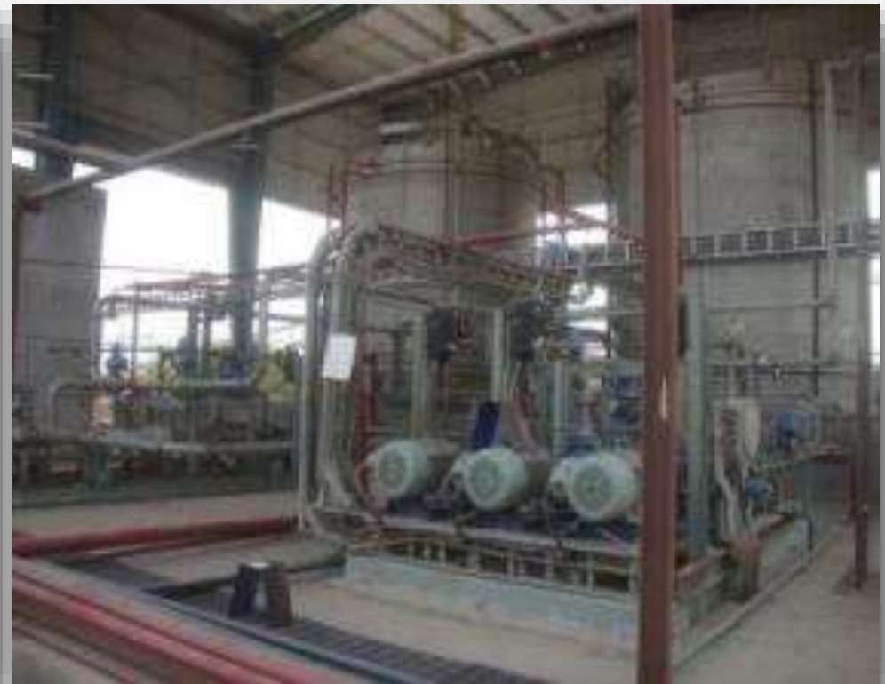
Solvent feed pumps
